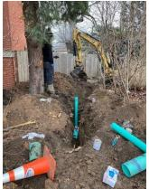
You may have noticed mounds of dirt along the Saratoga side of Crafts Hall and the sanctuary and the Harlem side of the sanctuary. Due to collapse and debris in the underground pipes that carry rain water from the Crafts Hall, Narthex, and Sanctuary roofs, rain water was leaking into the building and pooling on the floor in Youth Hall. During the week between Christmas and New Years 2021 a plumbing contractor dug trenches along
